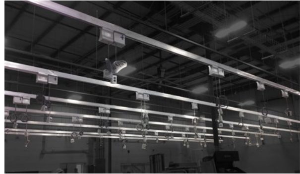
Figure 8. Conventional pipe & wire system (left) vs. track busway power distribution system (right)
